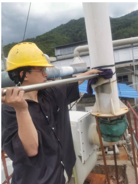
污水处理废气排气筒出口(FQPK-0005)G5
